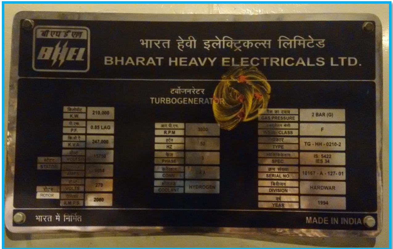
Figure:1 name plate details of 210 MW unit (BHEL Make)
